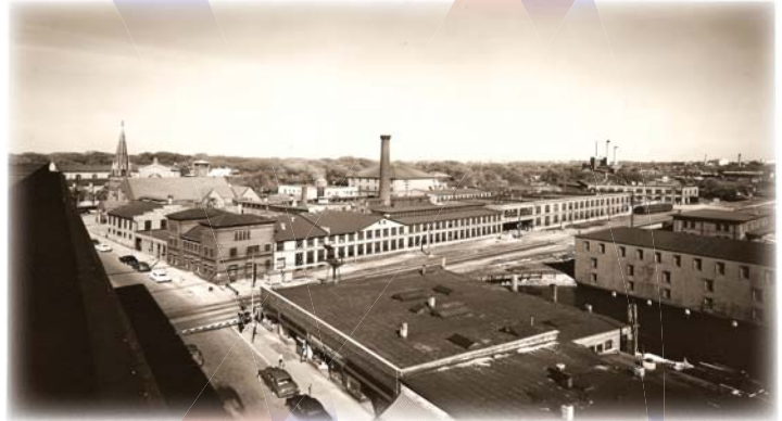
The original American-Marsh facility located in Battle Creek, Michigan, USA (Photo taken around 1950).
